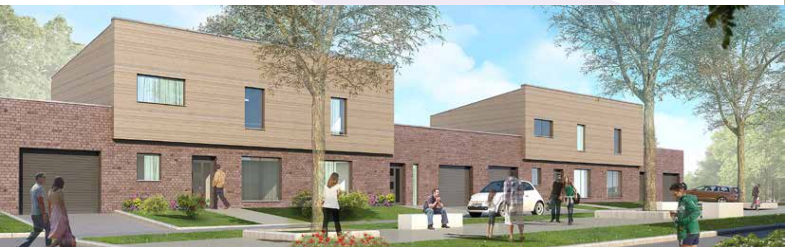
AULNOYE AYMERIES - 16 logements PSLA
